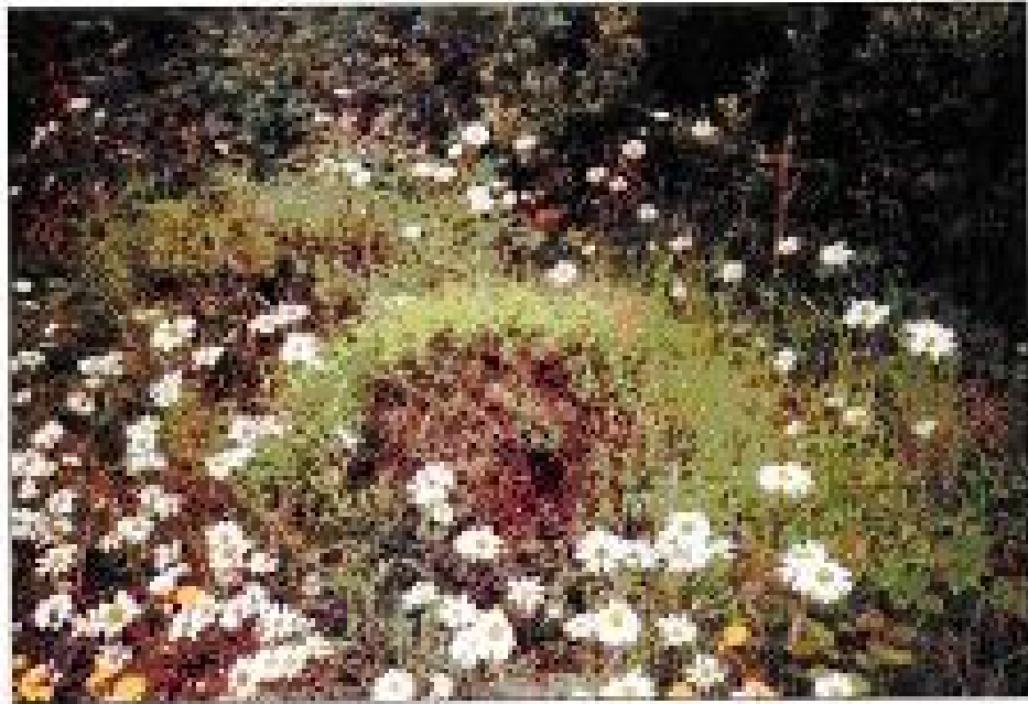
Photo 3 - Ant hill on embankment
