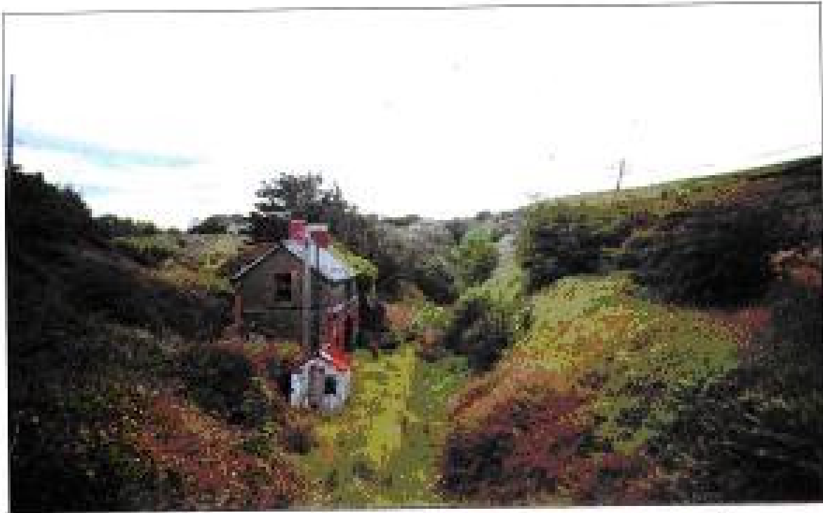
Photo 9 - Former station and shallow cutting, looking eastwards towards the tunnel.
