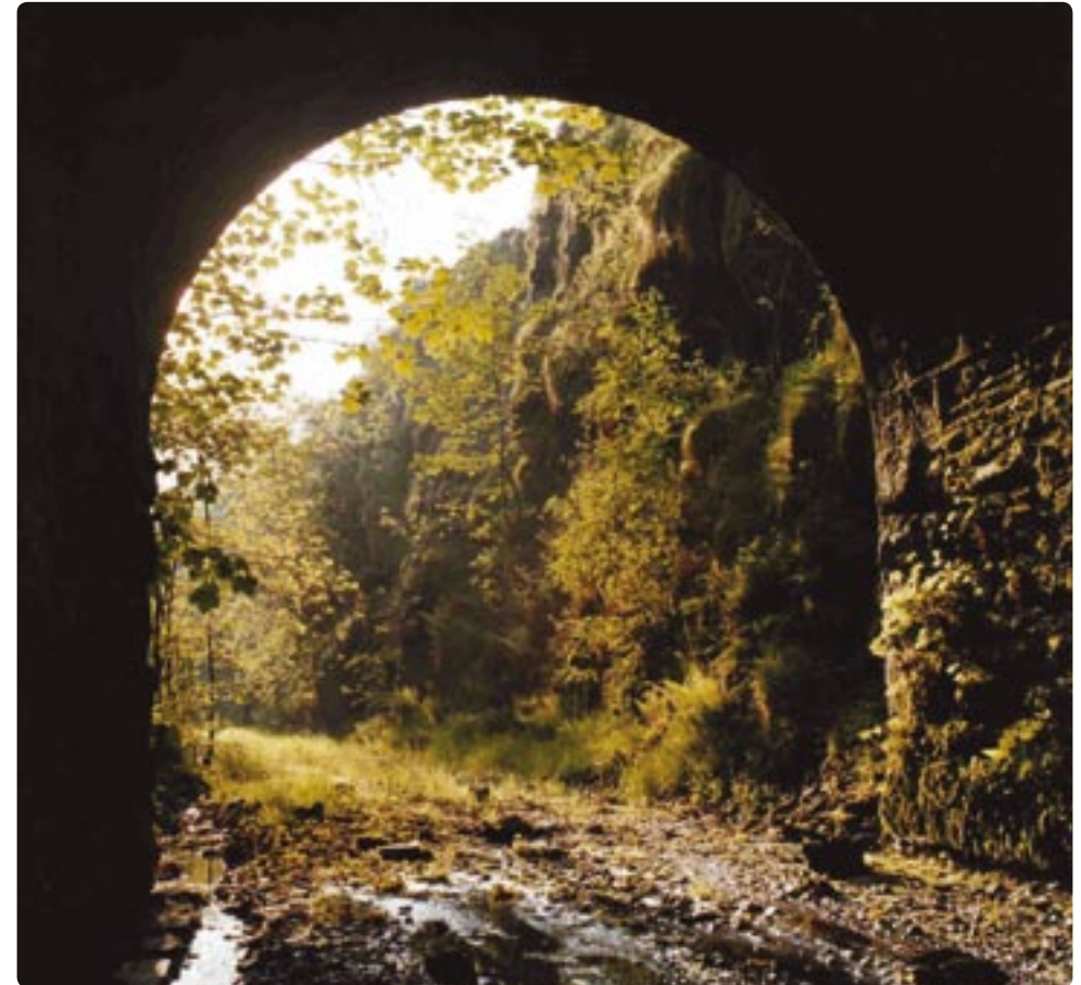
Barnagh Tunnel (John Considine)
